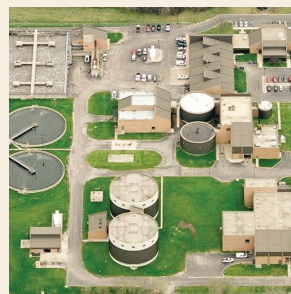
Woodridge Greene Valley Treatment Plant
