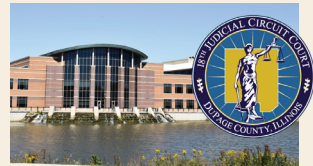
DuPage County Courthouse
